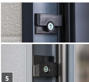
5 System preventing the leaf from dropping.
